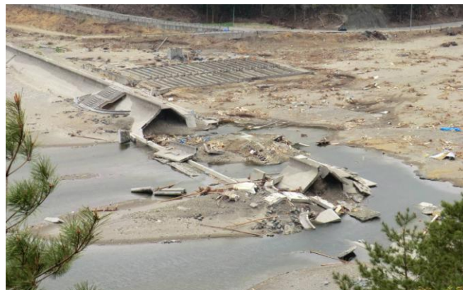
Figure 2. A typical coast fill-type dyke (Figure 1) that fully collapsed by tsunami, Aketo, Tanohara, Iwate Prefecture (by the courtesy of Prof. Koseki, J., Univ. of Tokyo)
